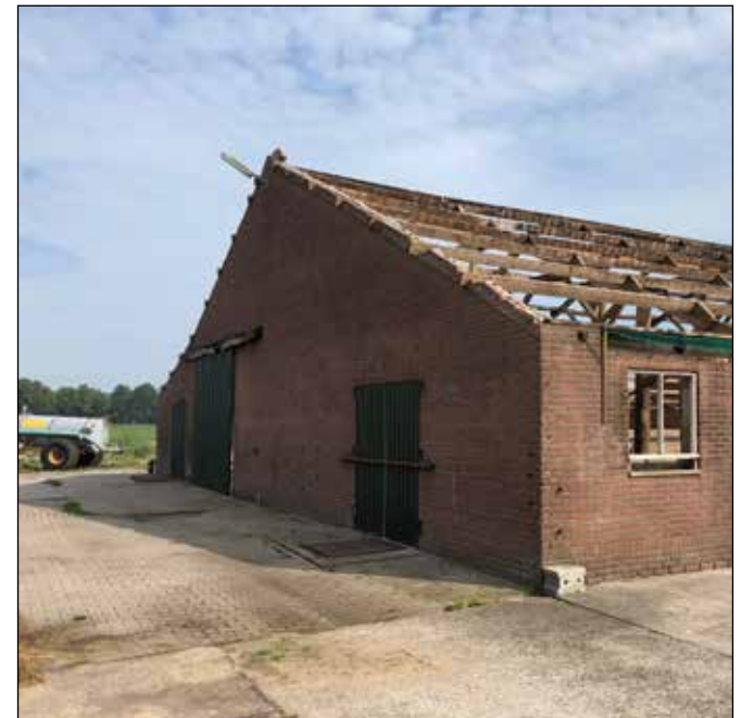
te slopen ligboxenstal
